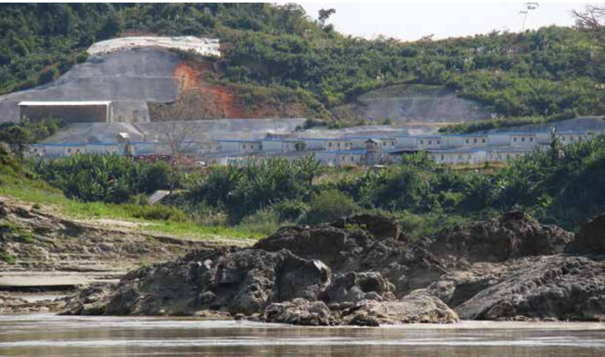
Myitsone Dam Site, Burma. If completed, Myitsone Dam would flood the confluence of the Mali and N'Mai rivers, which combine to create the mighty Irrawaddy River. The confluence is a spiritual and sacred place for the local Kachin people and the nation. Photo: International Rivers
